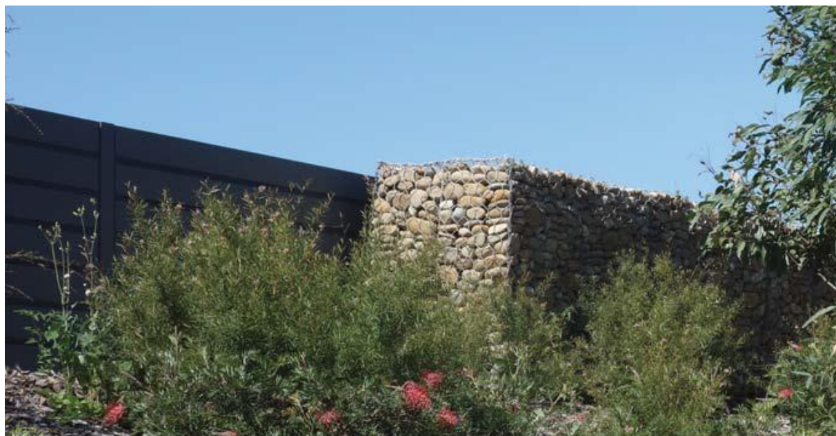
Figure 2-17: Indicative rock gabion and timber acoustic wall.
